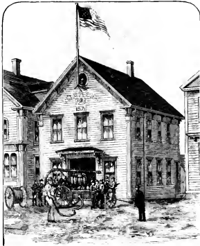
THE TORRENT ENGINE HOUSE. ERECTED IN 1874.
